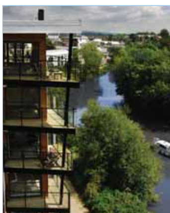
Contemporary riverside apartments
